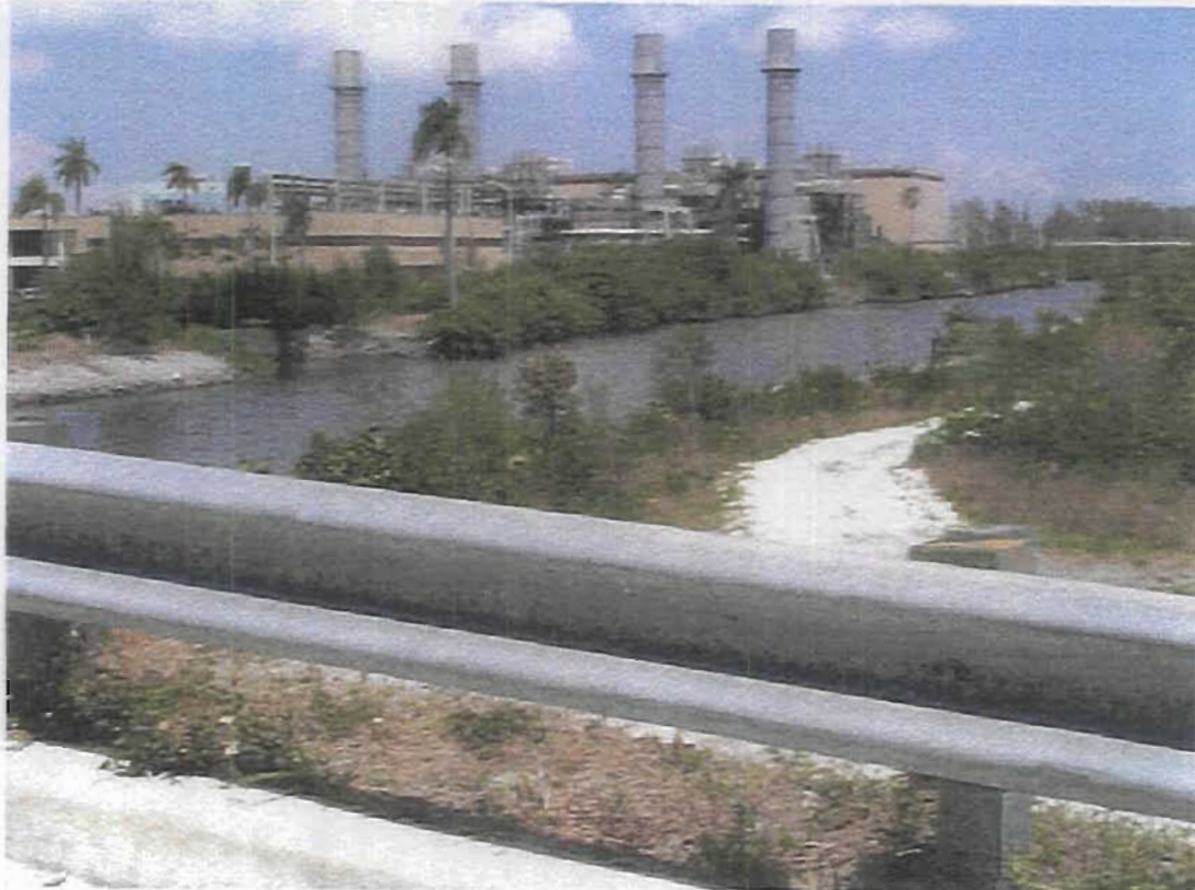
Figure 7 – View of Repowered FPL Lauderdale Plant
