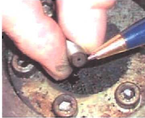
Figure 1-23 Plugged Distillate Fuel Orifice
