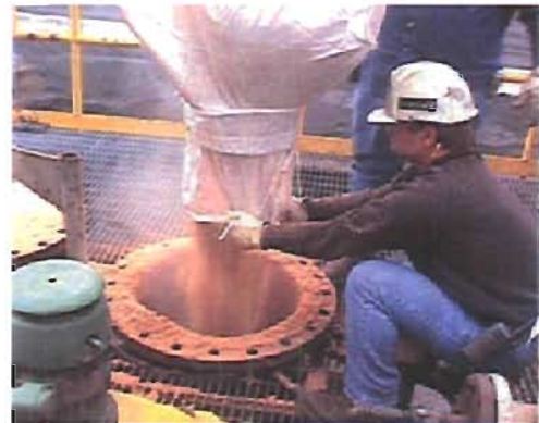
Emptying Totes Into Mixing Tank
