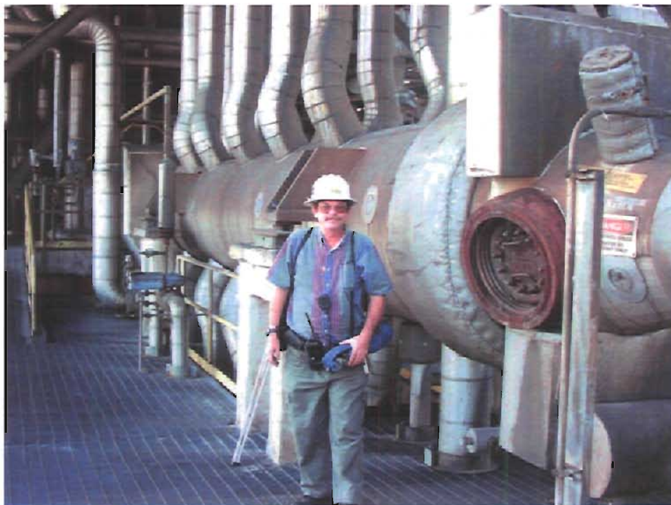
Figure 1-6 Convective Syngas Cooler Handhole Nozzle (Right) for Inspection and Some Cleaning of Outlet Tubesheet
