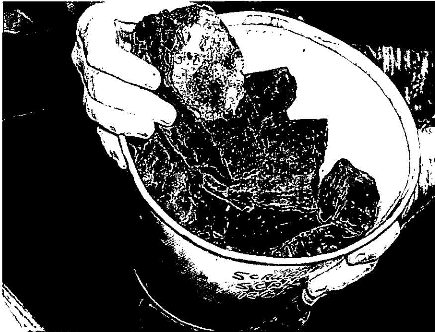
Figure 1-15 Hard 2 Inch Thick Scrubber Scale
