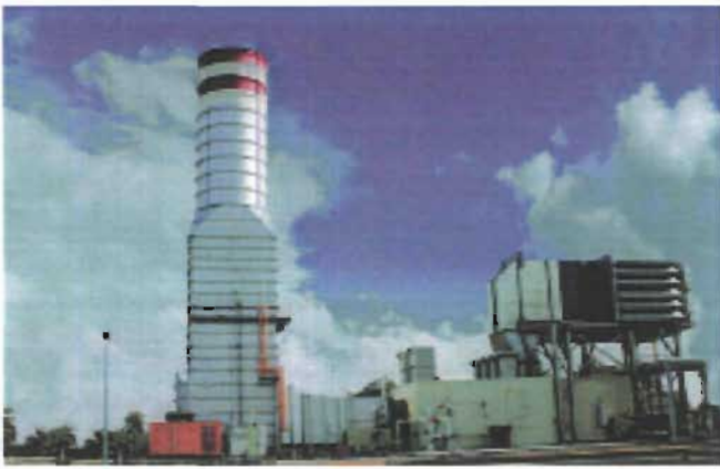
SGT6-PAC 5000F Power plant in typical arrangement
