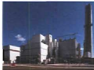
North County Resource Recovery Facility
