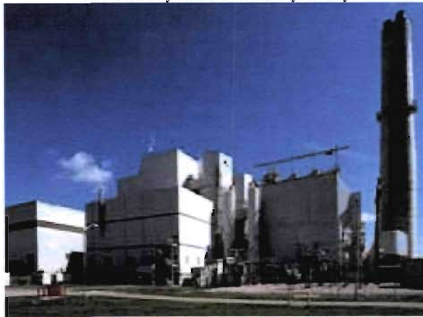
North County Resource Recovery Facility
