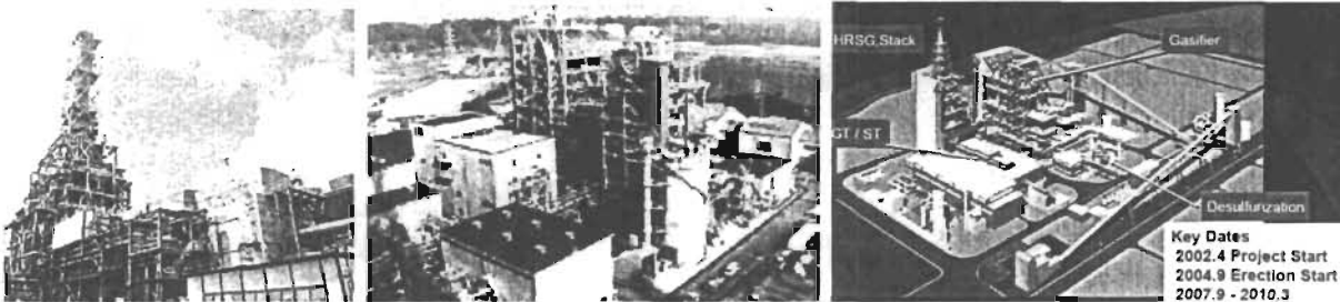
Figure 16. VR IGCC. Pilot & 250 MW Low Rank Coal-fueled, Air Blown, Slagging IGCC
