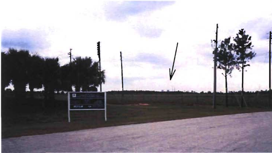
From the Orange County East Water Reclamation Facility (wastewater treatment plant), looking southeast.
