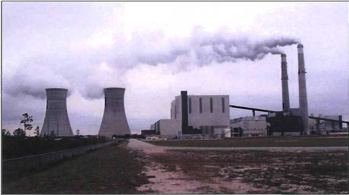
A. Existing power plant facilities (FLUCFCS 831)
