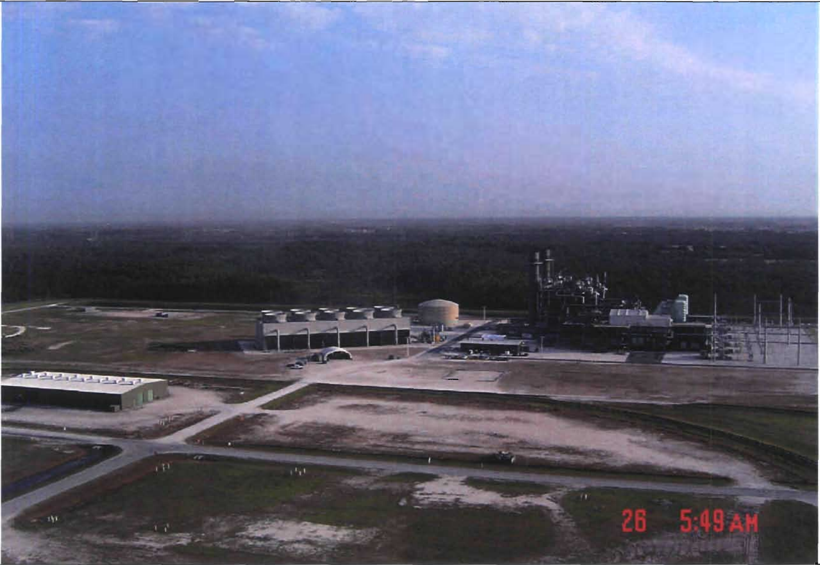
FIGURE 3.2-2. CURRENT VIEW OF PLANNED IGCC FACILITIES AREA
