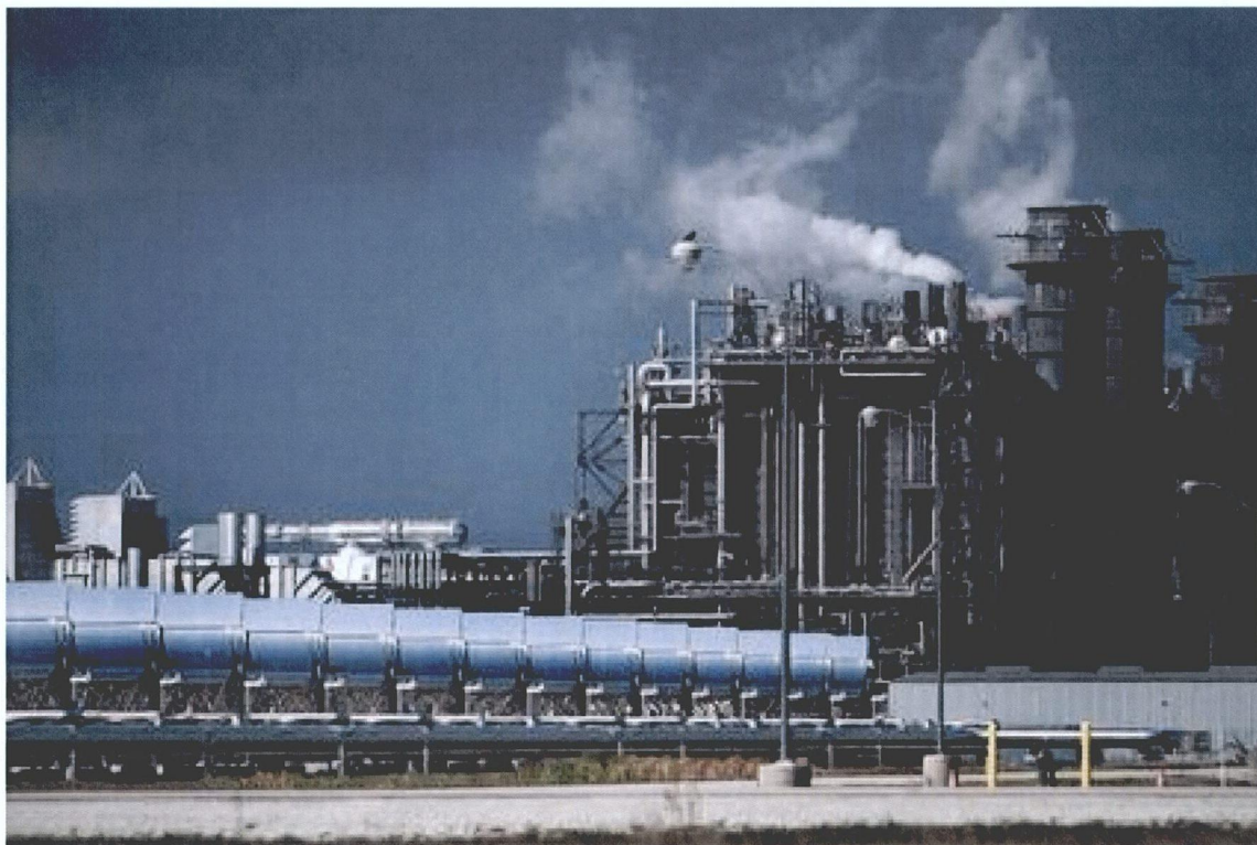
Figure 2. Unit 8 Inlet Filters on far Left. CT in the Middle. HRSG and Stacks on Right.
