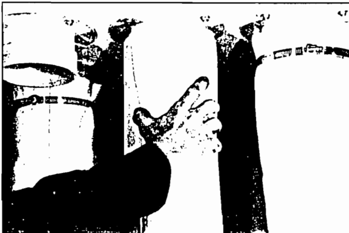
Step 3 The bag and cage are then slid onto the permanently attached bag cup.
