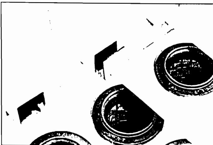
Step 5 The header pipes are easily installed by sliding the indexed end into the bracket.
