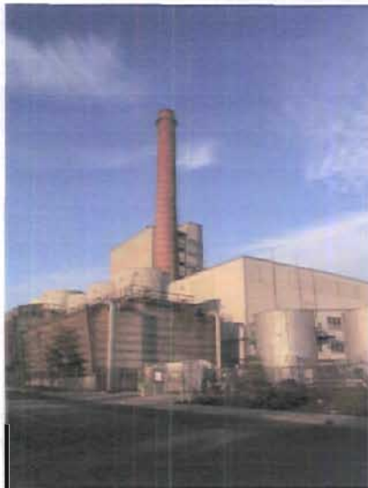
Figure 3 – J.R. Kelly Plant
