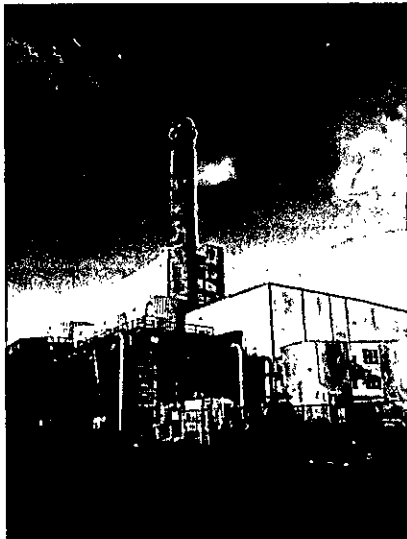
Figure 3 – J.R. Kelly Plant
