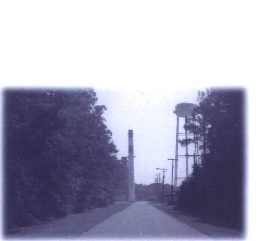
Entrance to the Sam O. Purdom Generating Station
