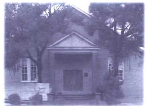
St. Marks Community Center
