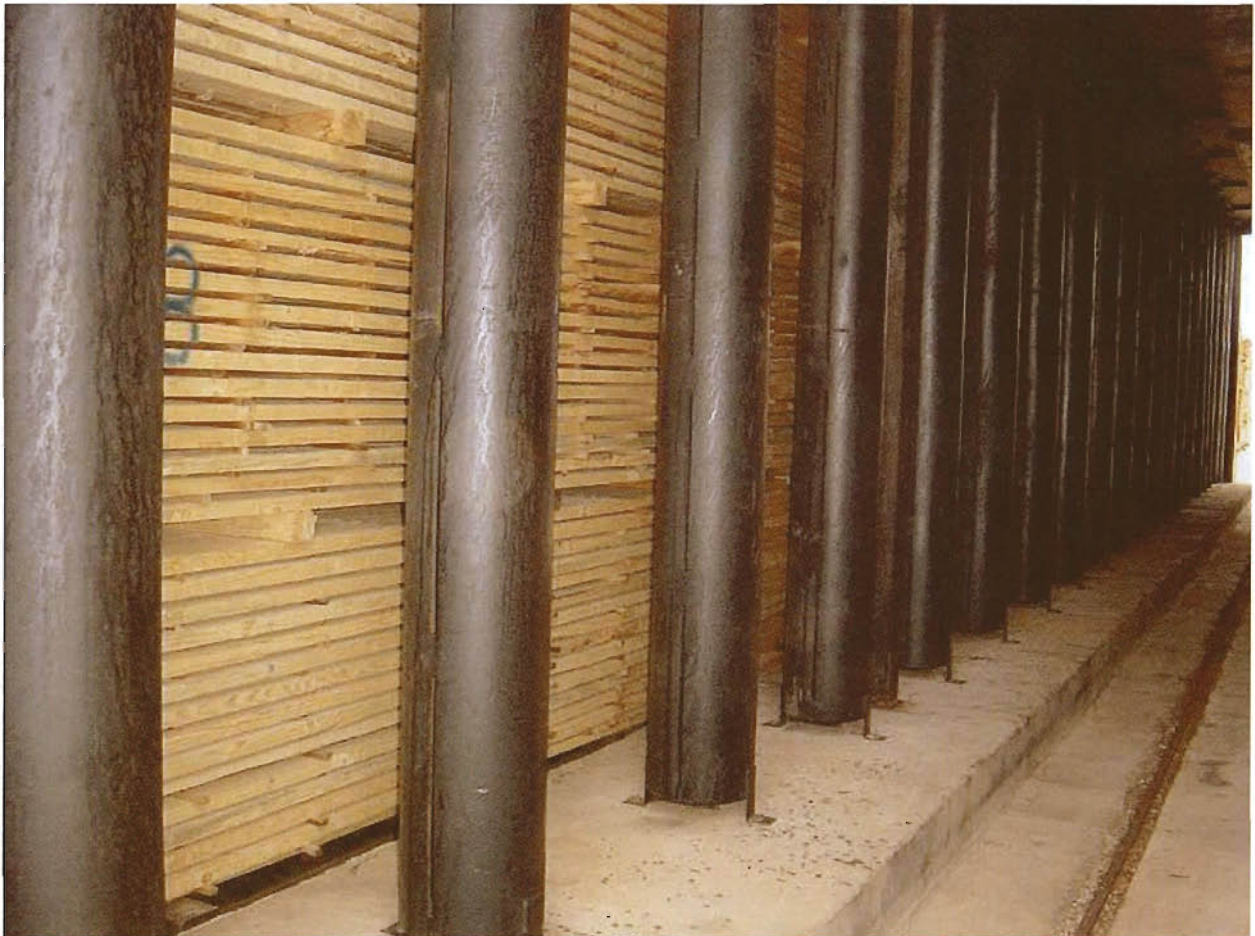
AERODYNAMIC DOWNCOMMERS PROVIDE REHEAT WITH MINIMAL AIR FLOW DISRUPTION
