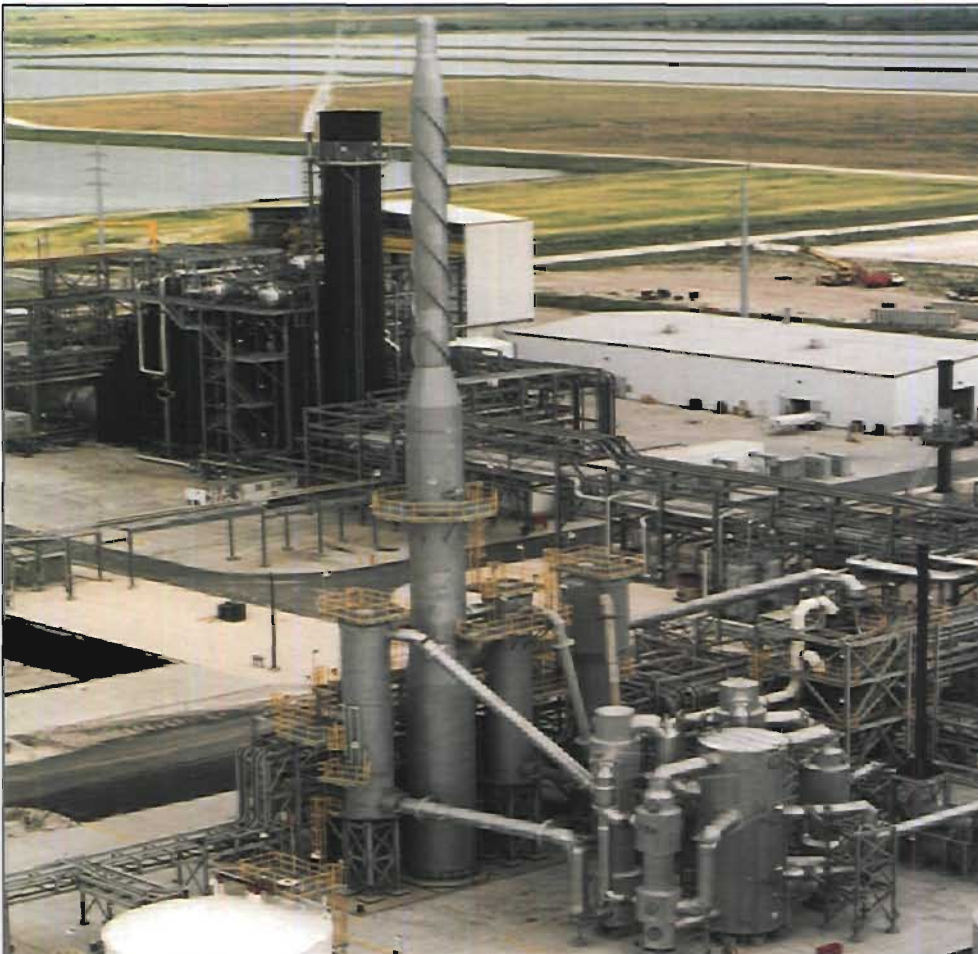
The sulfuric acid plant is in the foreground and the combined-cycle unit is in the background. The large black object (left center) is the heat recovery steam generator.
