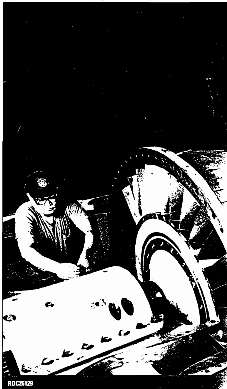
▲ The stator incorporates six major sections, split in half for easy maintenance.
