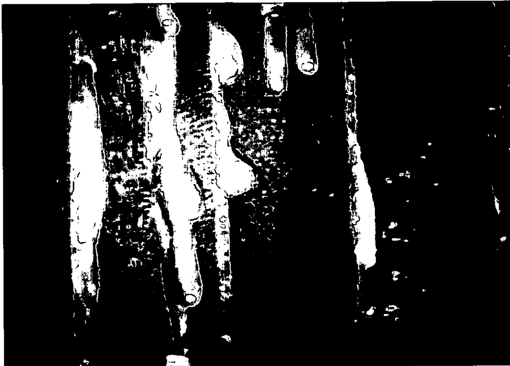
Close-up of deposits in HRSG, low-pressure section of economizer.
