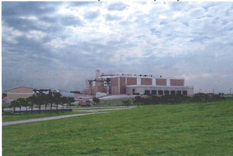
Pinellas County Resource Recovery Facility
