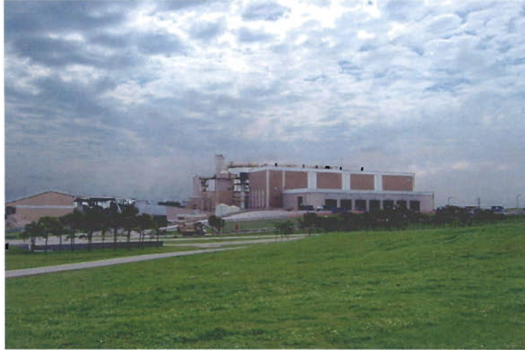
Pinellas County Resource Recovery Facility
