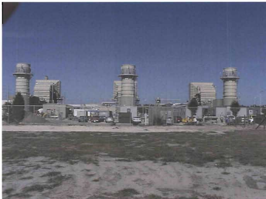
Photo 2. Front View - Combustion Turbine
