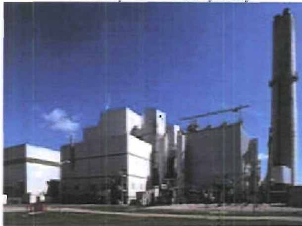
North County Resource Recovery Facility
