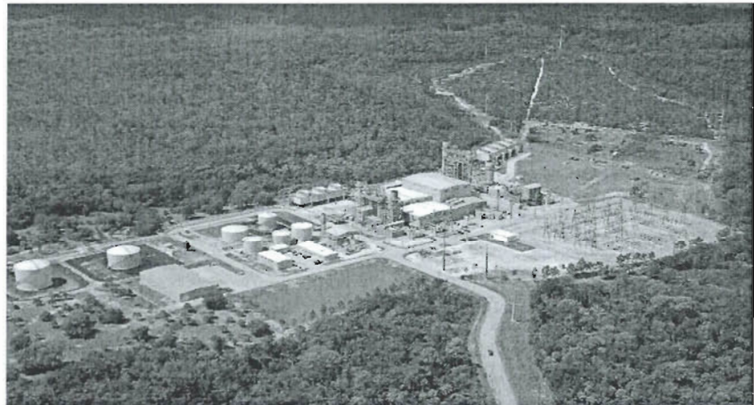
Figure 2. Aerial View of CIPP Units 1, 2 and 3 (left to right)
