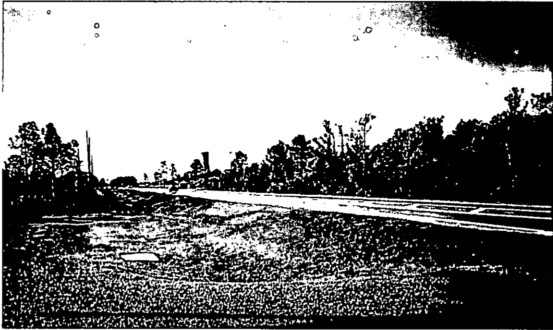
FROM THE ENTRANCE TO AVALON PARK OFF ALAFAYA TRAIL, LOOKING SOUTHWEST.
