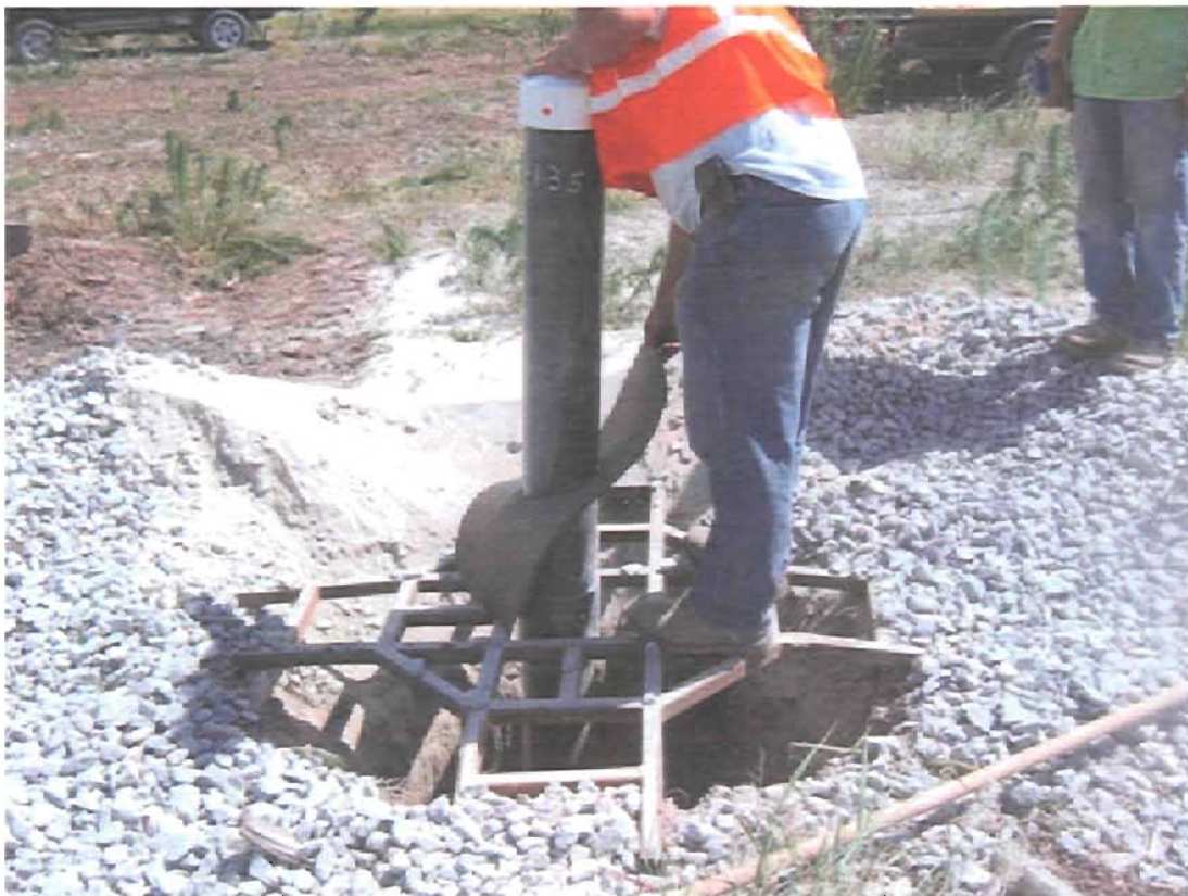
FIGURE 4: Installing the geotextile pad.
