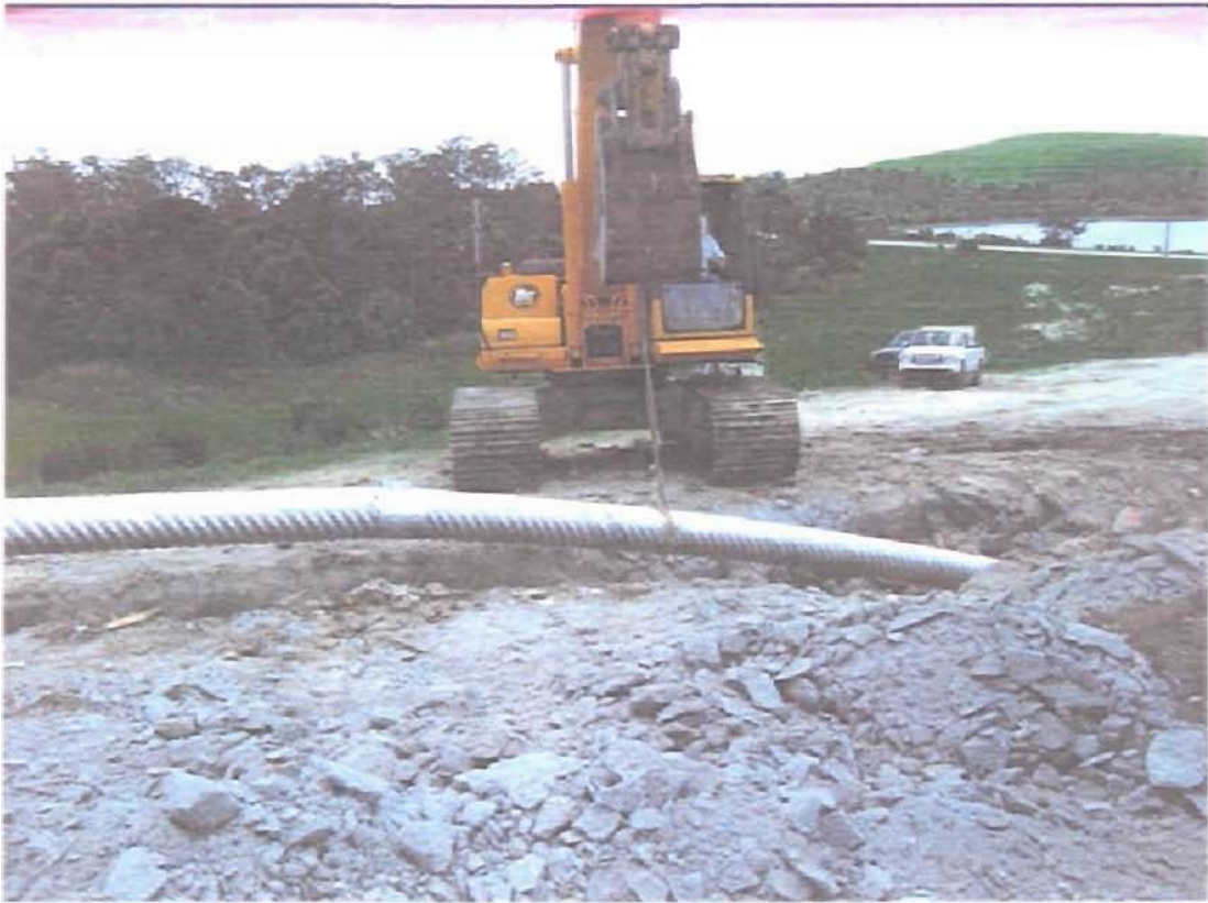
FIGURE 9: Laying CMP under the access road.
