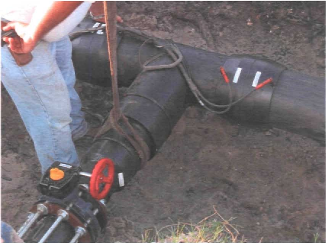
FIGURE 7: Using electrofusion couplings to fuse a lateral onto the header pipe.
