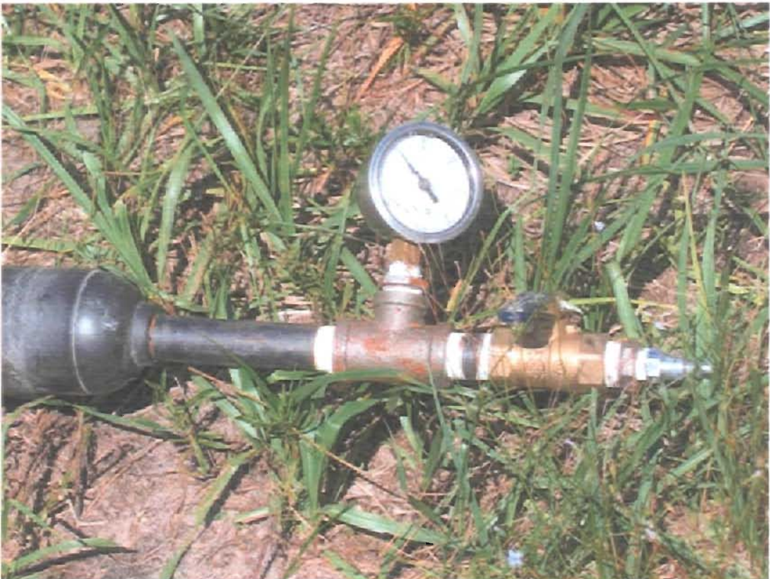
FIGURE 8: Pressure testing a lateral.
