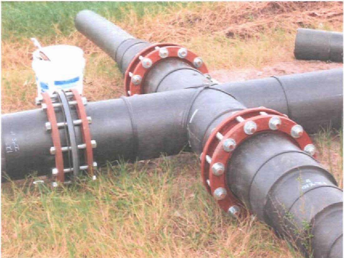
FIGURE 10: Fabricating the condensate knockout.
