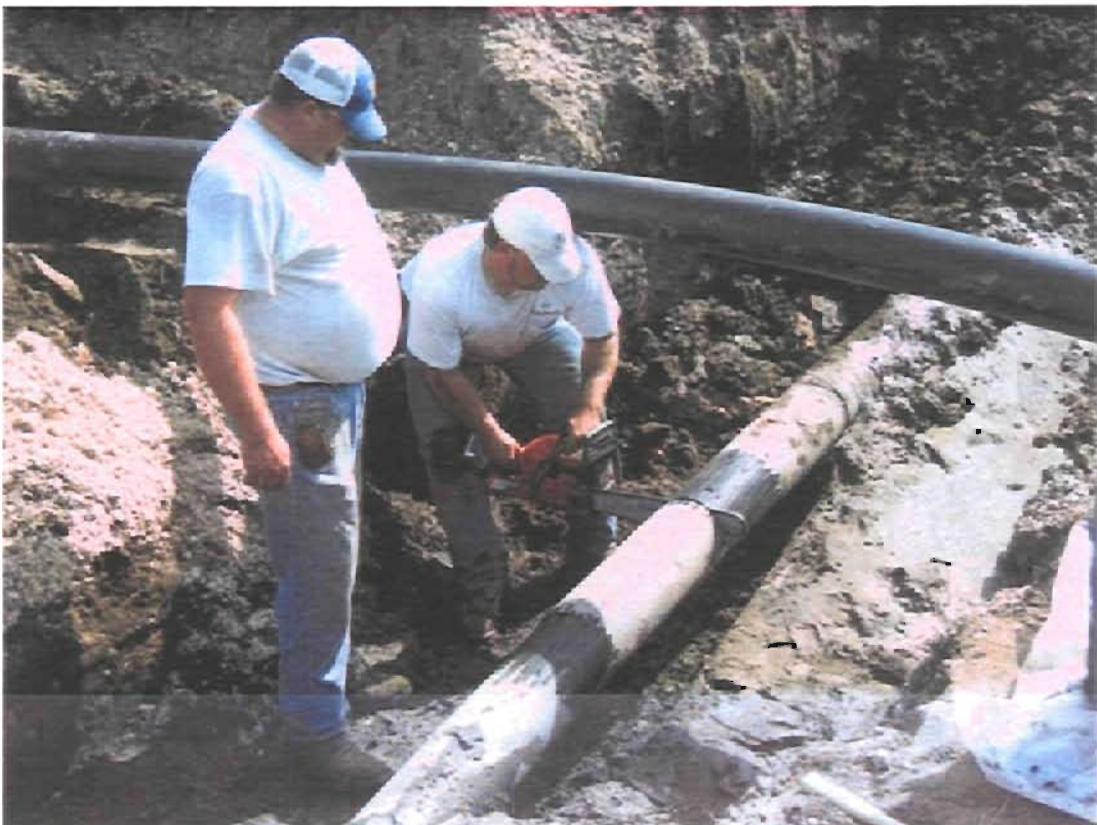
FIGURE 6: Cutting a header to fuse a lateral onto the header pipe.
