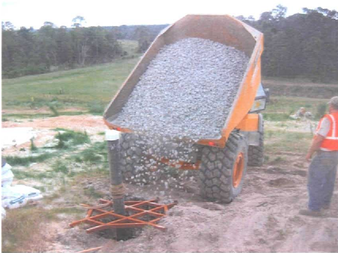
FIGURE 3: Filling the borehole with rock to 1' above the perforated section.
