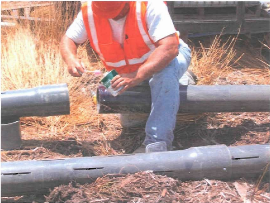
FIGURE 2: Gluing a section of solid pipe to the perforated pipe.
