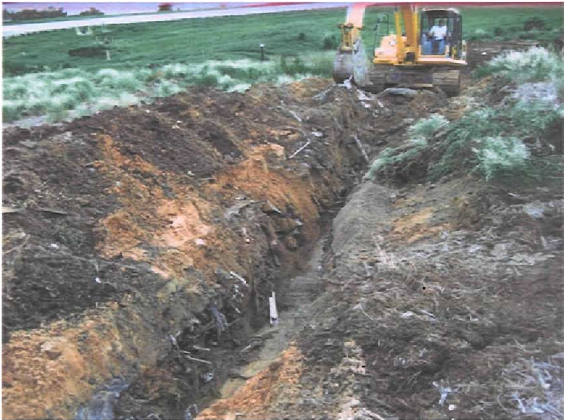
FIGURE 5: Trenching to lay the laterals.
