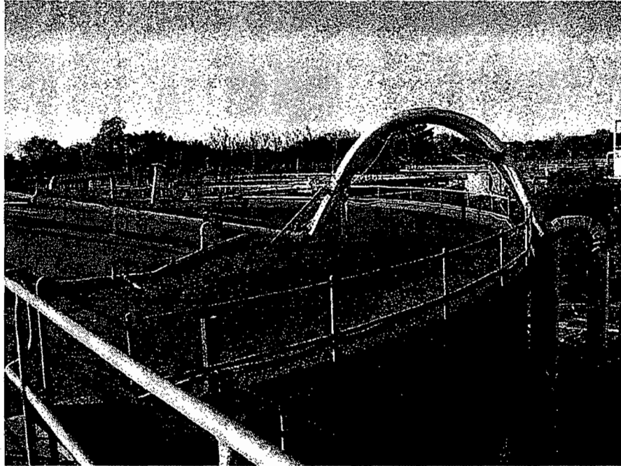
Photograph 1: Digester No. 6 Gas Collection Piping
