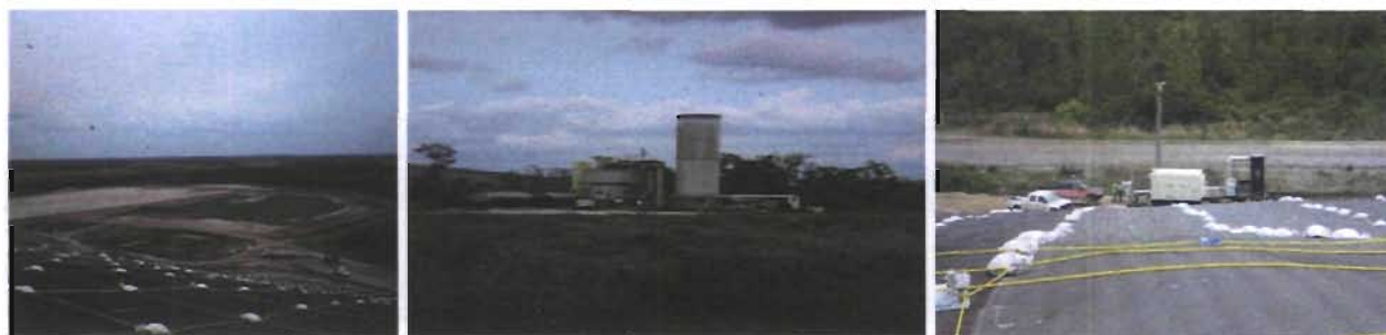
Figure 7 – Berman Landfill Figure 8 – Existing Enclosed Flare Figure 9 – Temporary Odor Flare
