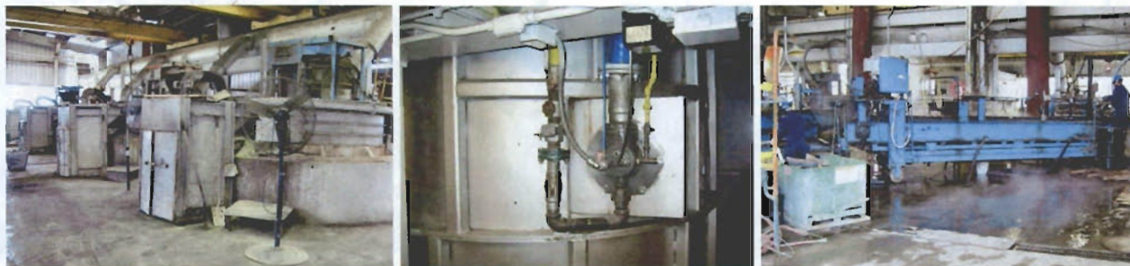
Figure 12. Refining kettles and ducts, gas burner on kettle at GRC, ingot casting machines.
