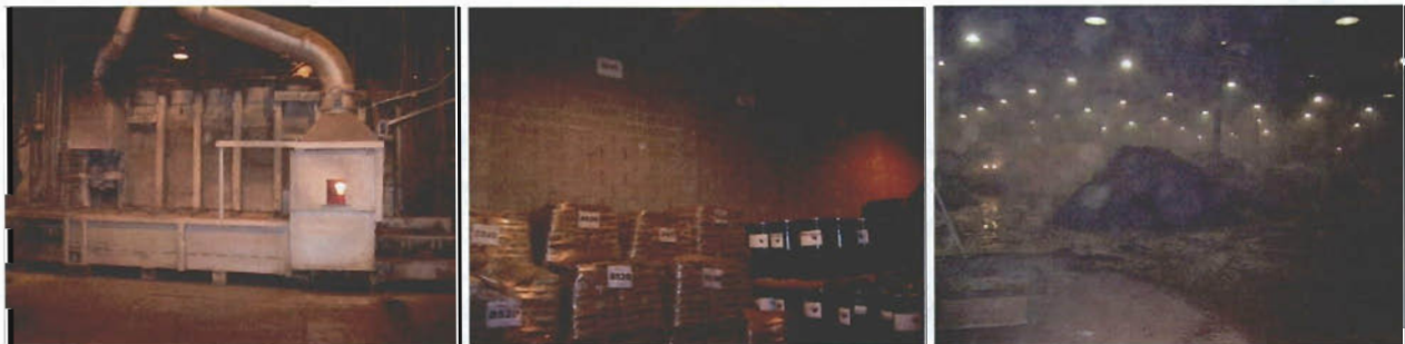
Figure 16. Reverb furnace, chemical storage, totally enclosed raw materials storage area.
