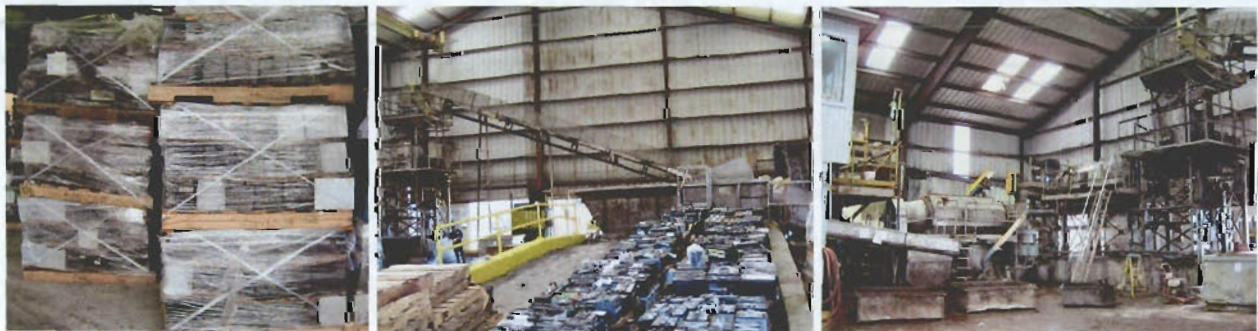
Figure 6. Received lead batteries, staging and conveyance, hammer mill and wet screening.
