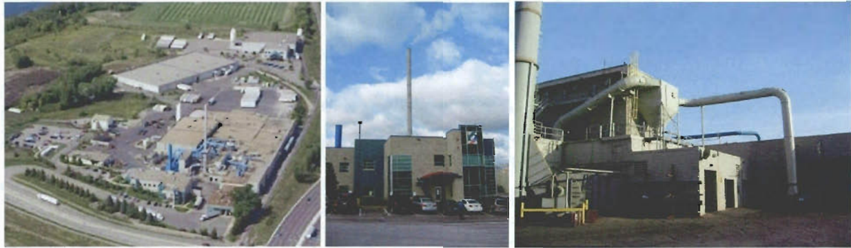
Figure 17. Overview of GRC, office building, enclosed operation, good ducts and baghouses.
