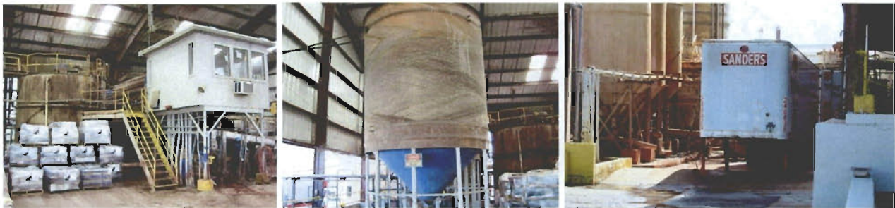
Figure 7. Settling tank & control room, sulfuric acid storage, trailer awaiting load of plastics.
