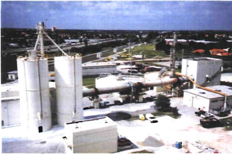
Figure 3-1 Alexander Orr, Jr. WTP Lime Recalcining Plant
