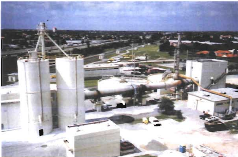
Figure 3-1 Alexander Orr, Jr. WTP Lime Recovery Plant
