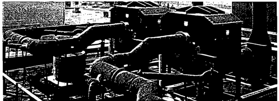
Two 9000 cfm roof-mounted Whirl Wets at BASF Wyandotte, Holland, MI.
