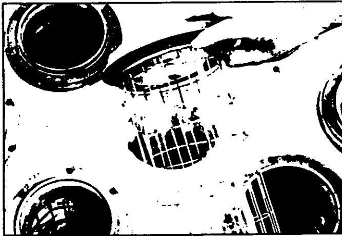
Step 3 Snap band with high profile lip seals secure the bag to the tube sheet.
