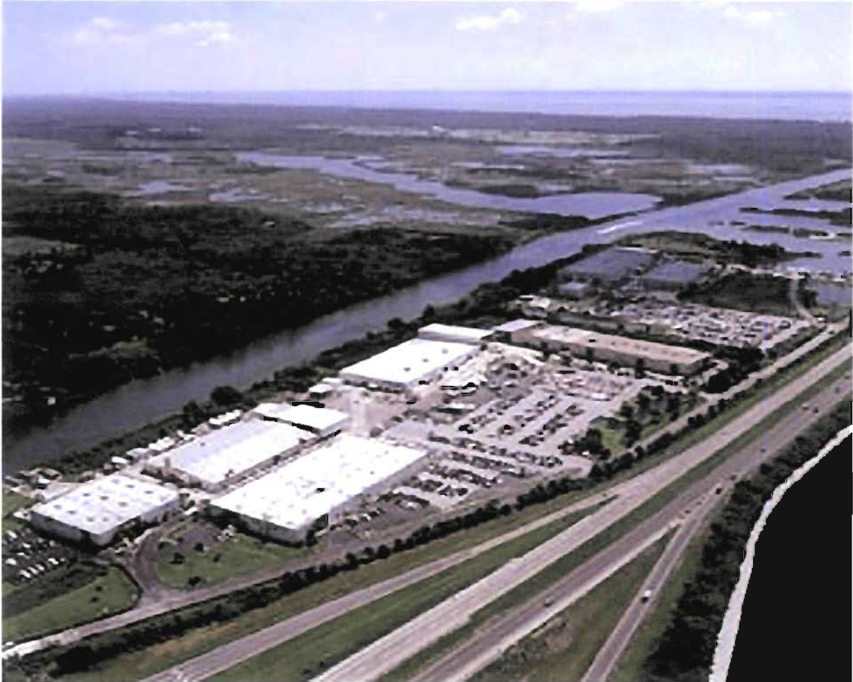
Figure 2. Aerial View of Developed Facility (Source: www.searay.com )
