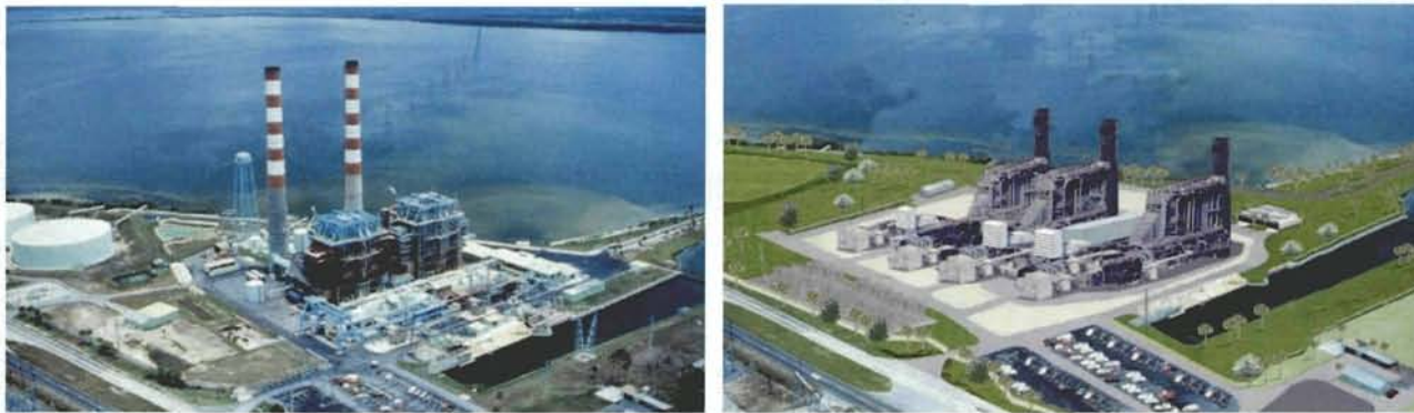
Figure 2. FPL Cape Canaveral Units 1 and 2. Artist Rendition of New Combined Cycle Unit
