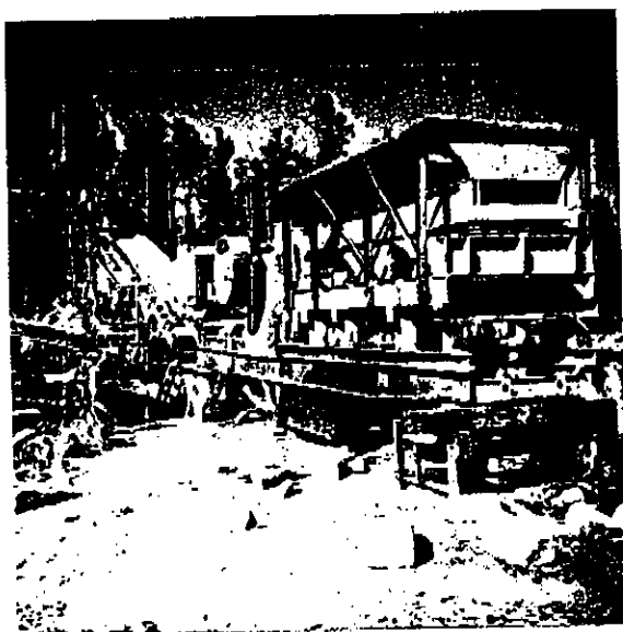
Mullinix Rock Crusher at AC Campment 11/7/00 Jaw crusher near shaker deck 12:30pm
