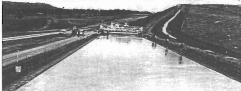
ROLLER COMPACTED CONCRETE
