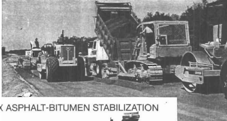
SOIL CEMENT - CEMENT TREATED BASE
