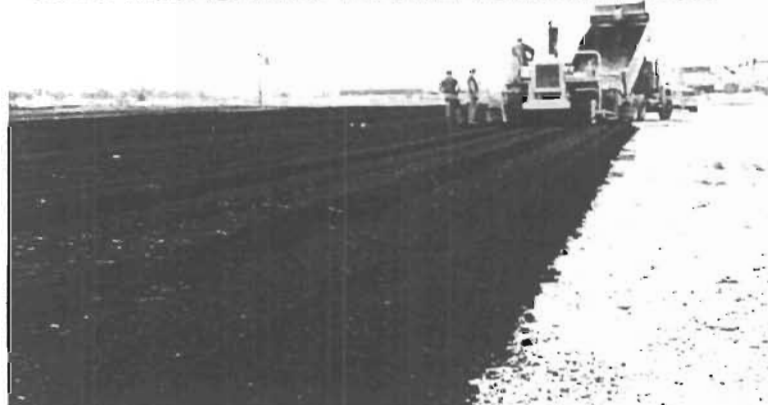
COLD MIX ASPHALT-BITUMEN STABILIZATION
