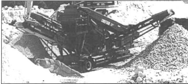
Direct-feed Chieftain 510 screening lime rock in Miami, FL
