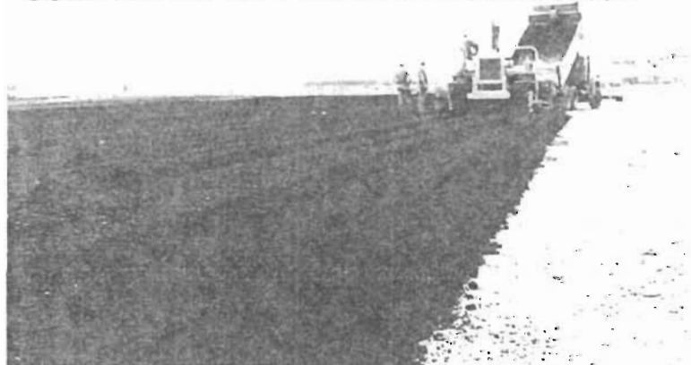
COLD MIX ASPHALT-BITUMEN STABILIZATION
