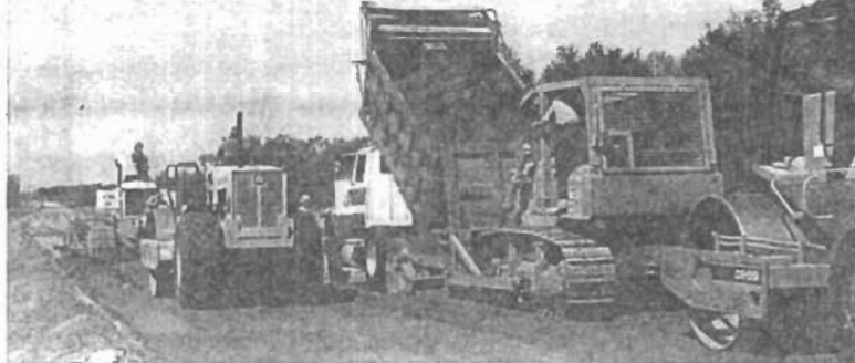
COLD MIX ASPHALT-BITUMEN STABILIZATION
