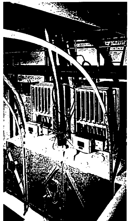
Compact — Two Dalmatic DLM-V6/10B insertables installed in a factory producing plastic bottles.
