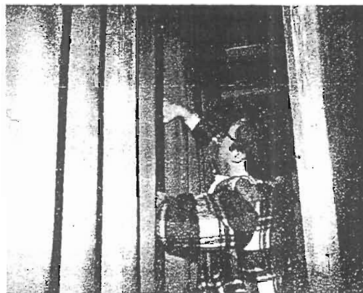
Figure 20. Inspecting shaker baghouse bags.
