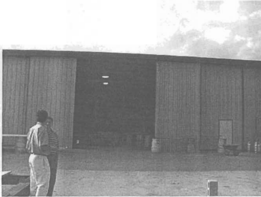
Photo 1 Existing "new" Facility with Full Height Door
