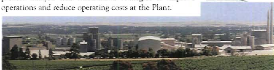
The Angaston Division of Adelaide Brighton Cement Ltd. Australia.
