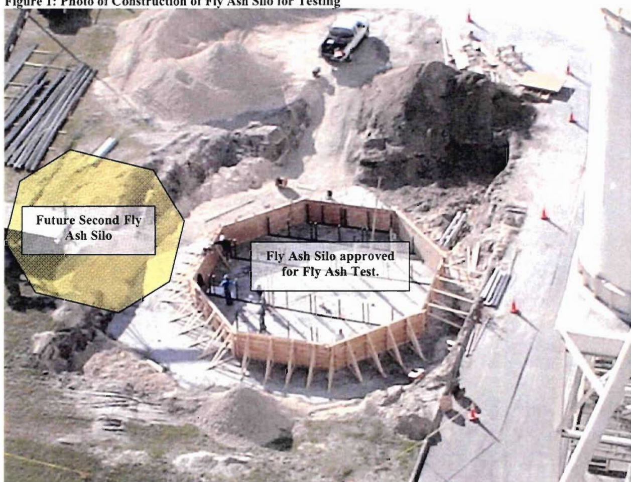
Figure 1: Photo of Construction of Fly Ash Silo for Testing
