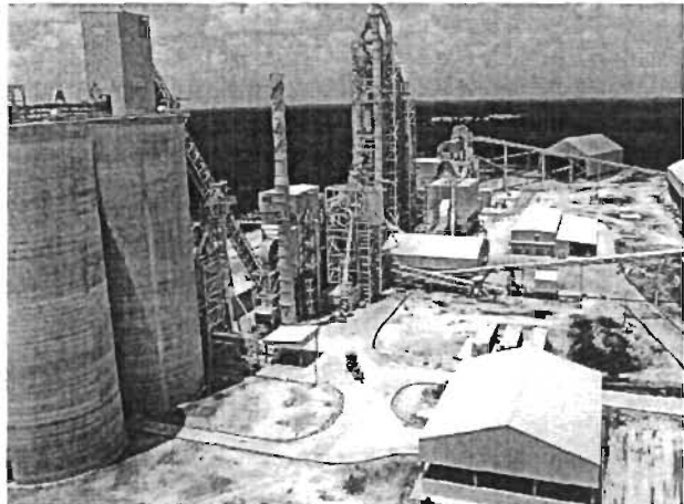
Completed Cement Plant (Photo SAC Website)
