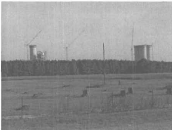
Cement Plant Under Construction (Photo DEP)
