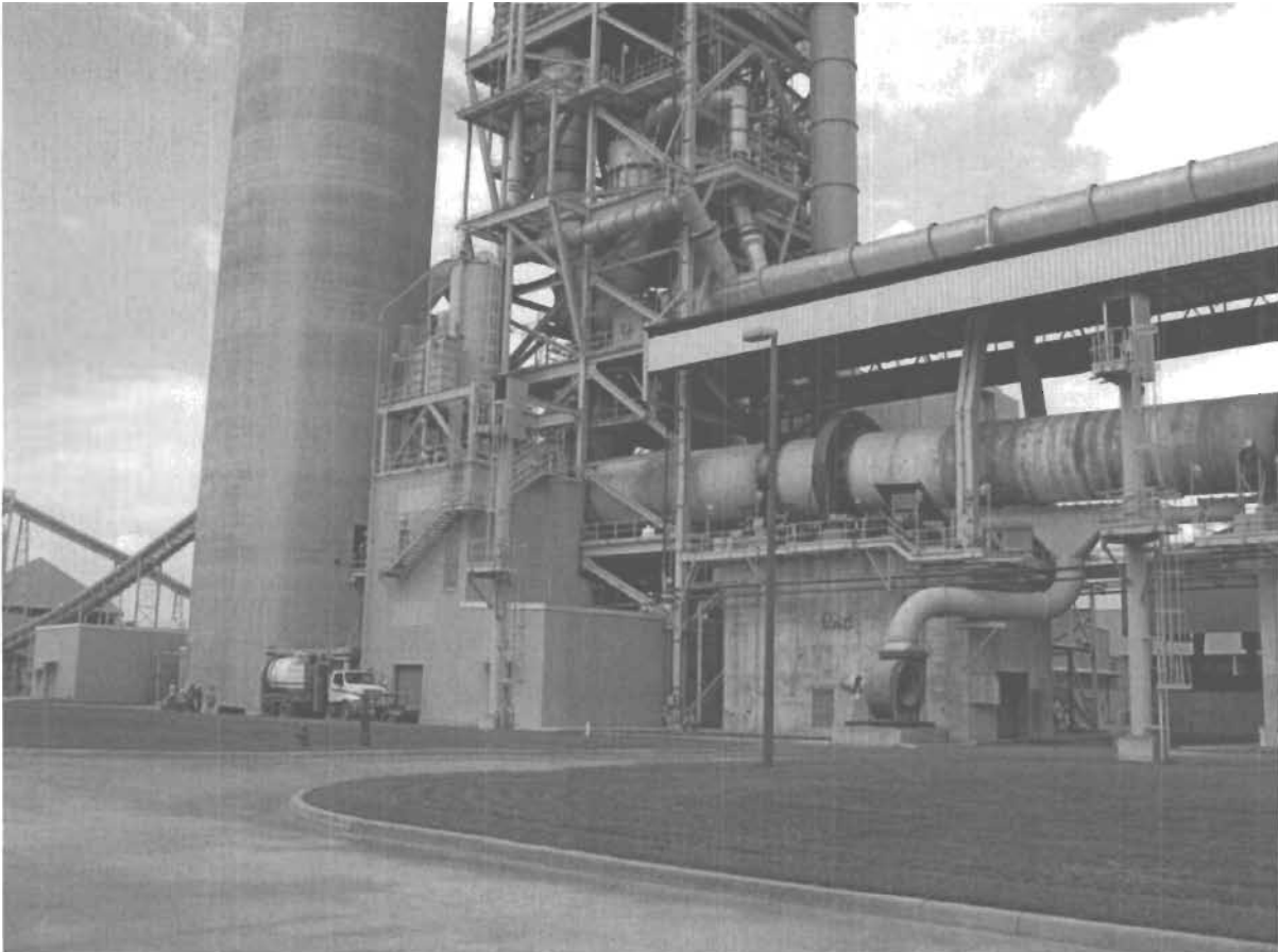
Kiln Inlet, Main Stack, Lower Preheater, Calciner, and Tertiary Air Ducts (Photo A. Linero)
