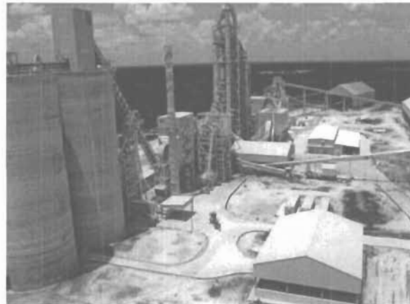
Completed Cement Plant (Photo SAC Website)
