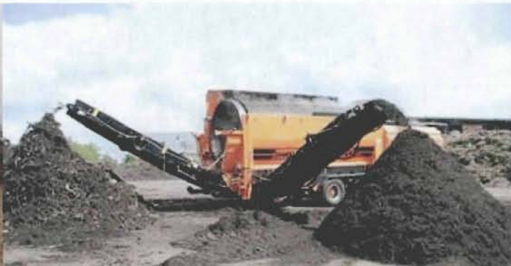
Figure 2.3 Image of a Doppstadt mobile screen in operation.
