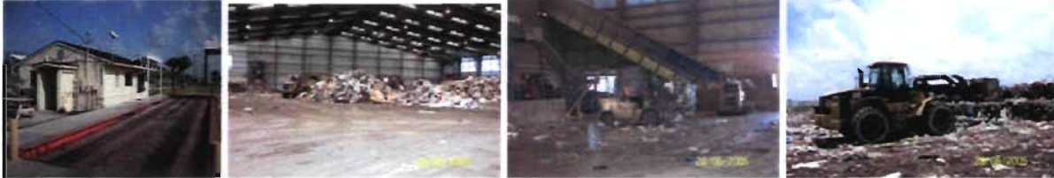
Figure 3. Scale House, Tipping Floor, Baling Room, Outdoor Bale Stacking at “Balefill”
