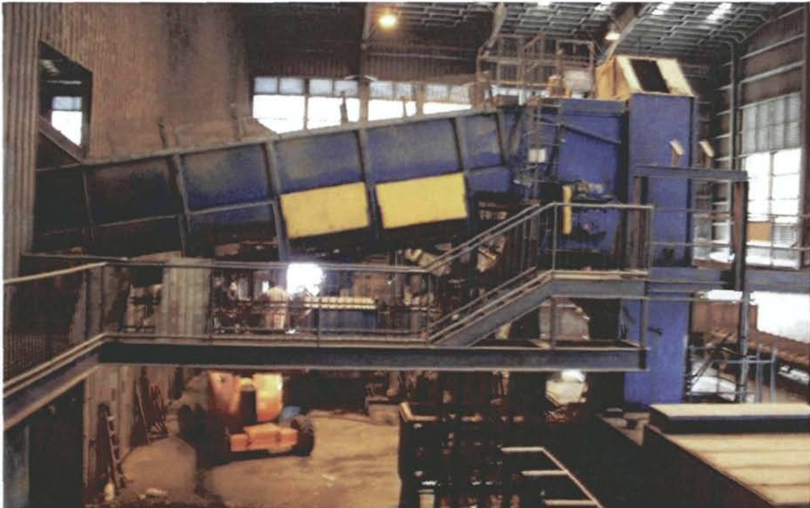
Figure 5. Existing Balers in Baling and Receiving Building
