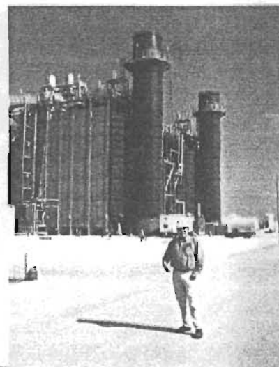
Figure 10 – Hines Power Block 1
