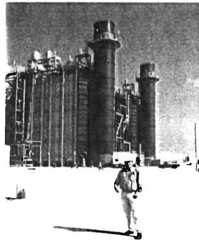
Figure 10 – Hines Power Block 1
