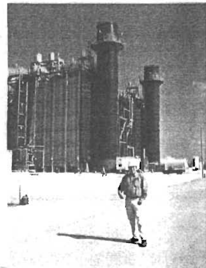
Figure 10 – Hines Power Block 1
